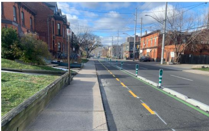
Hunter St, Hamilton Flexposts and precast curbs
