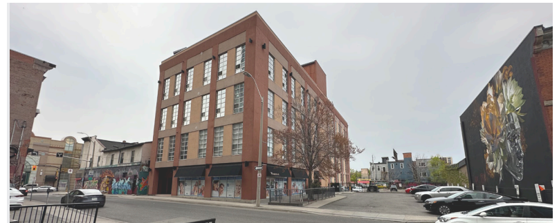
Figure 9. Existing buildings along Rebecca Street
