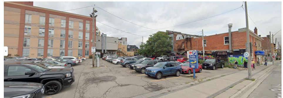
Figure 4. Northwest view of Subject Site from Hughson Street North
