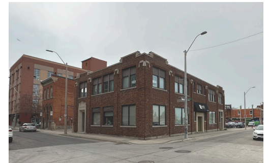
Figure 12. Existing buildings at Hughson Street North and Rebecca Street
