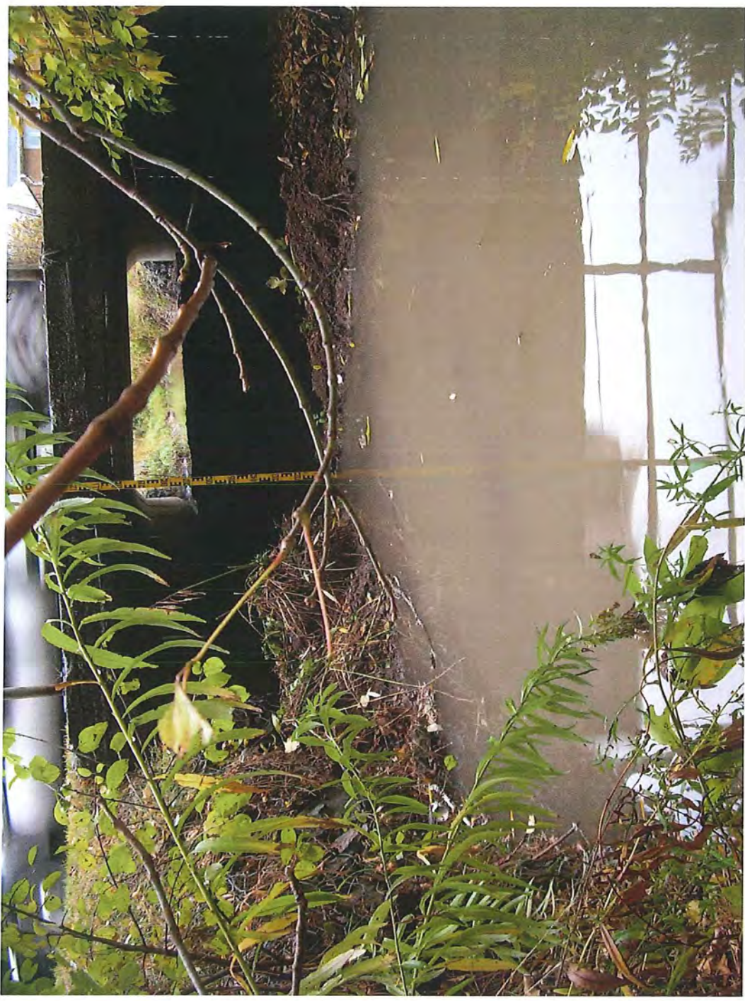
Photo 5: Watercourse 5, Arvin Ave crossing (downstream looking south)
