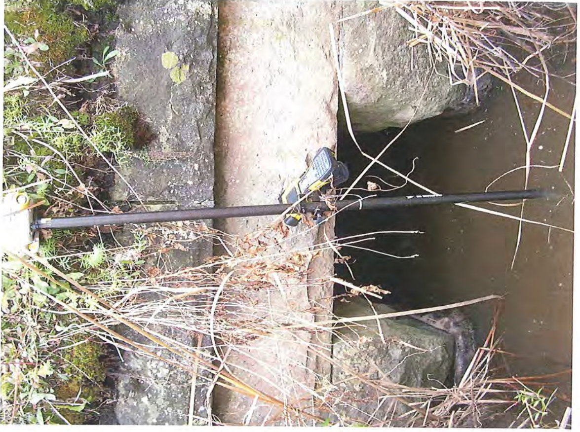
Photo 39: Watercourse 6.1, CN Rail crossing (downstream looking south)
